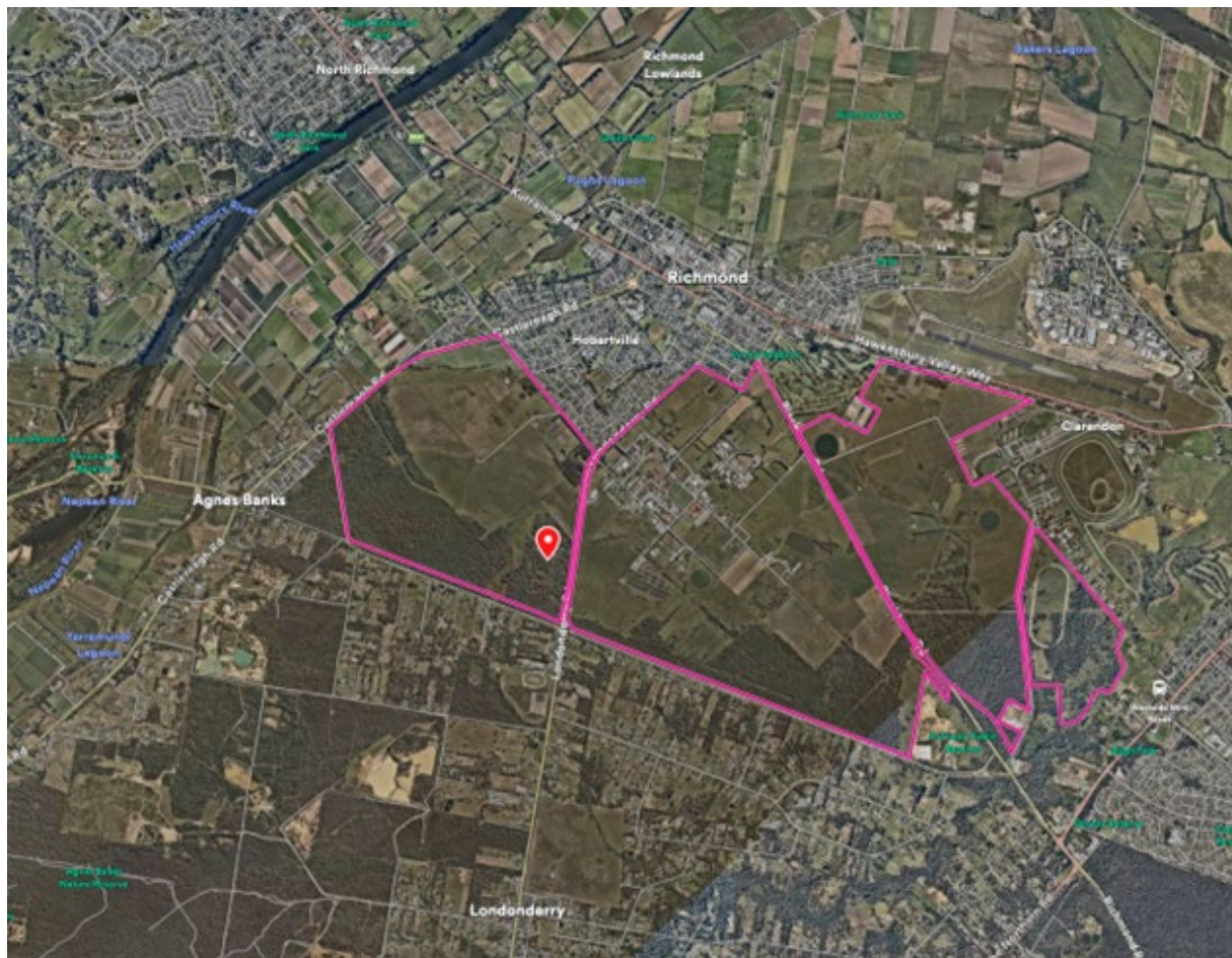
Figure 1: Hawkesbury campus – showing bushland works site
