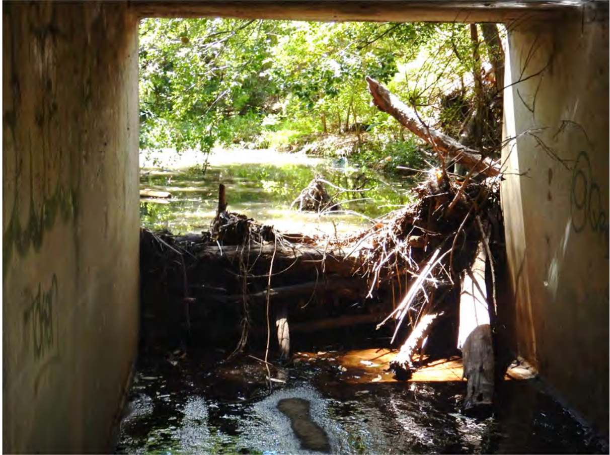
Plate 7. Debris blocking the rail bridge culvert within Vineyard Creek on the eastern extent of the subject site
