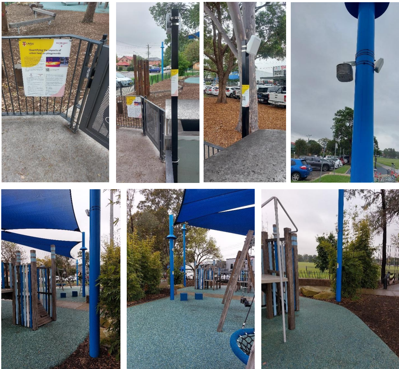
Figure 9. Sensors installed at Doyle Ground.
