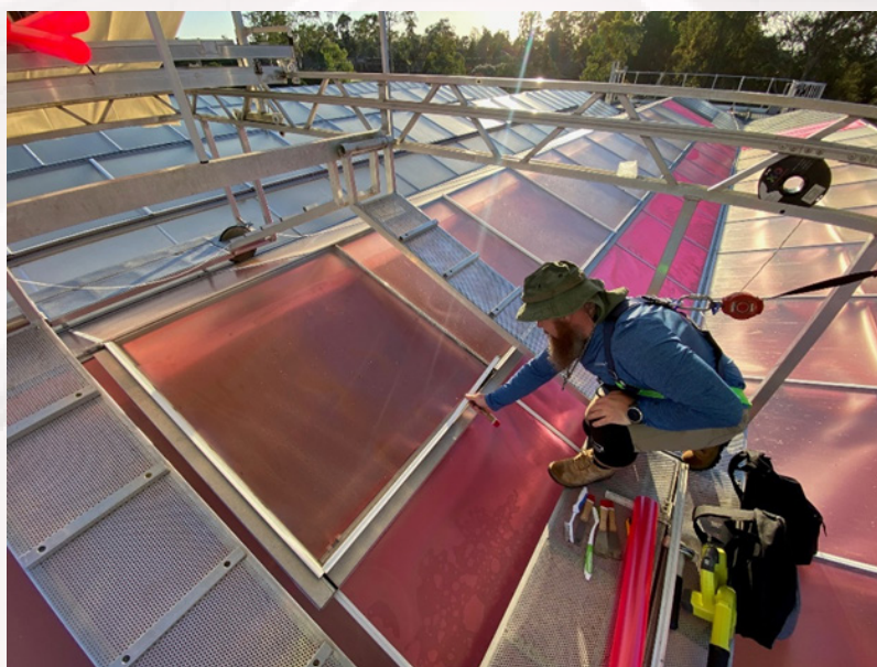
Image: Technical Assistant, Norbert Klause, installing Smart Film above S40
