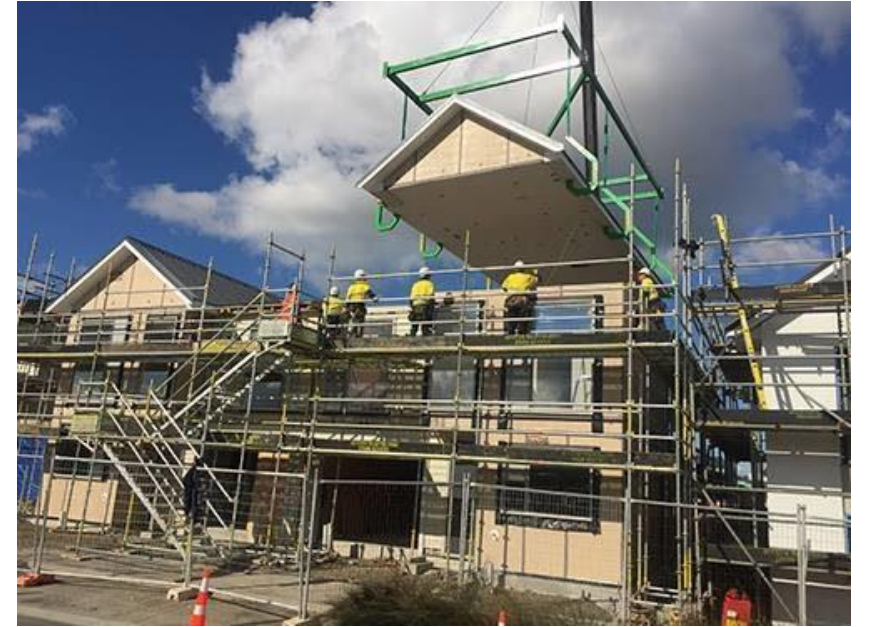
On site assembly of prefabricated elements at Hobsonville Point
