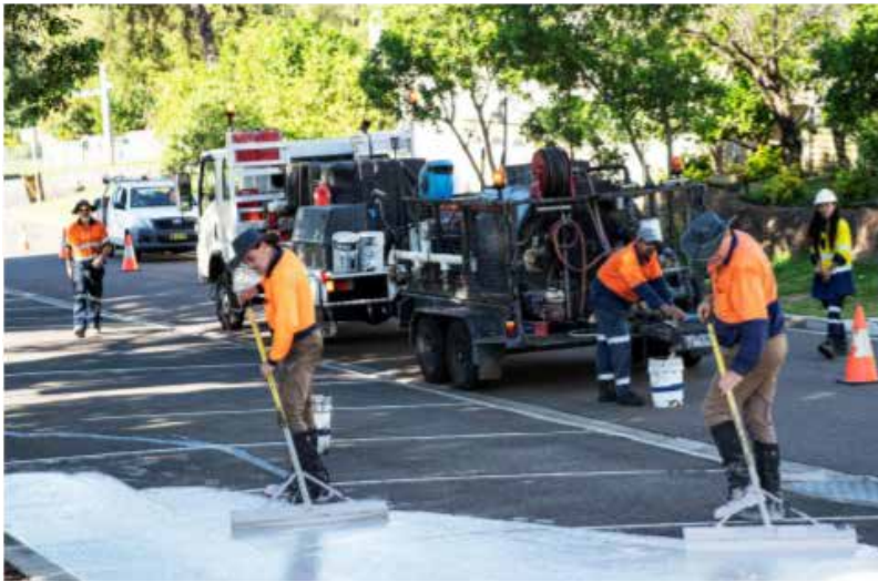
FIGURE 19: Cool Roads Trial 2021. The left image shows the application of the reflective surface paint. The right-side graph shows the cooling potential of the coated surfaces is larger when surfaces get hotter. © George Gittany.
