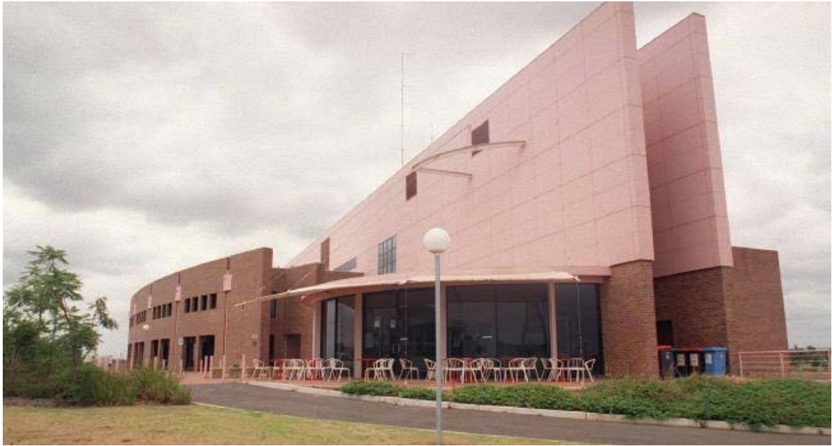
Picture – Front of Building BA
