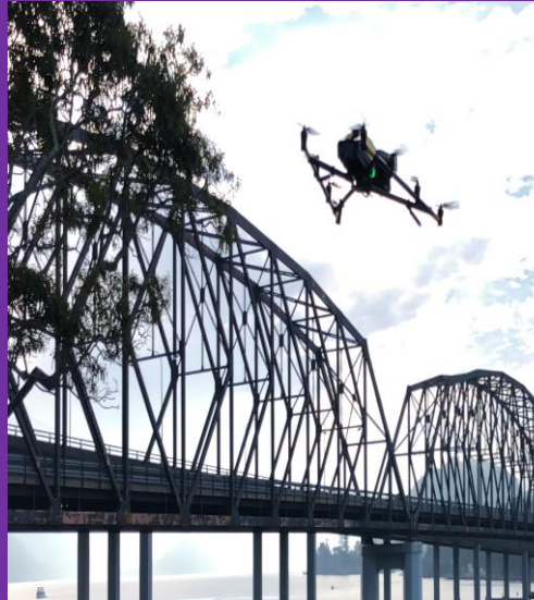
Assessment of Peats Ferry Bridge using Intel Falcon 8+ Drone
