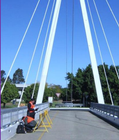
Structural Assessment and Health Monitoring of Werrington Bridge
