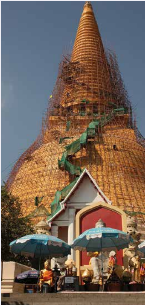
Phra Pathom stupa in Thailand under renovation in 2010
